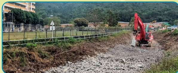
移除東涌河渠道化河床 Removal of the channelised riverbed of Tung Chung Stream
