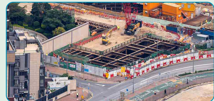
西污水泵房現正進行鋼筋混凝土結構工序 The reinforced concrete works at the West Sewage Pumping Station are in progress
