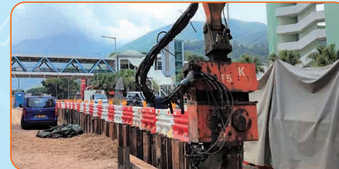
於松仁路的中央分隔帶進行板樁工程 Sheet piling works at central median of Chung Yan Road are in progress
