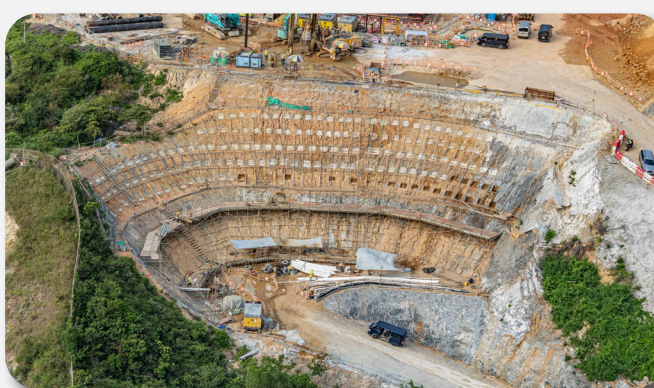
於斜坡進行泥釘建造工程 Installation of soil nails on the slope
