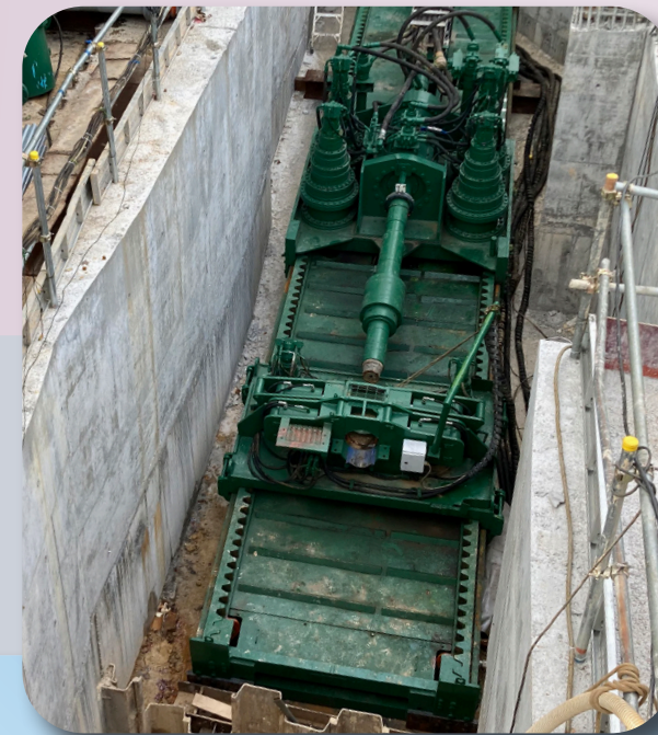
定向鑽掘法為全陸地鑽掘式的非開挖工程技術 HDD is a surface-launched, remotely controlled drilling technique
