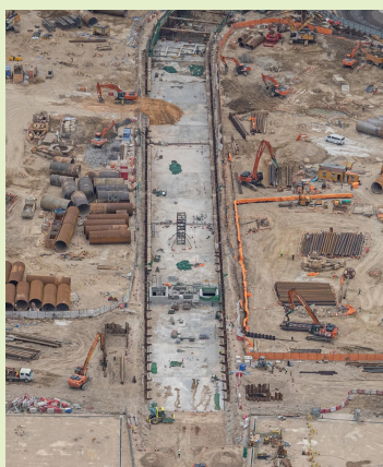
建造箱型排水暗渠 (航空照片) Construction of box culvert (aerial photograph)
