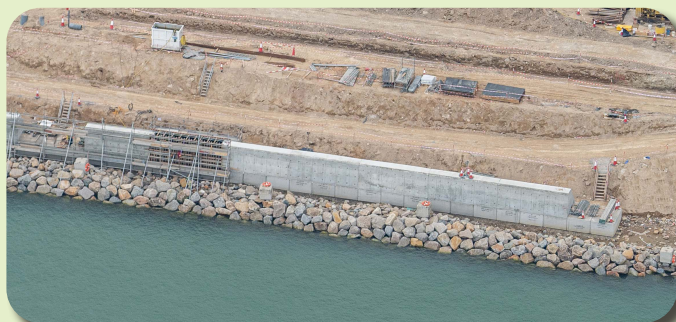
建造海堤 Construction of seawall
