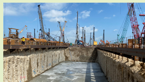
利用深層水泥拌合法形成的擋土牆 Retaining wall formed by DCM method
