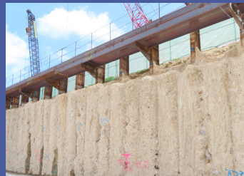
STAGE 1: Installation of DCM
